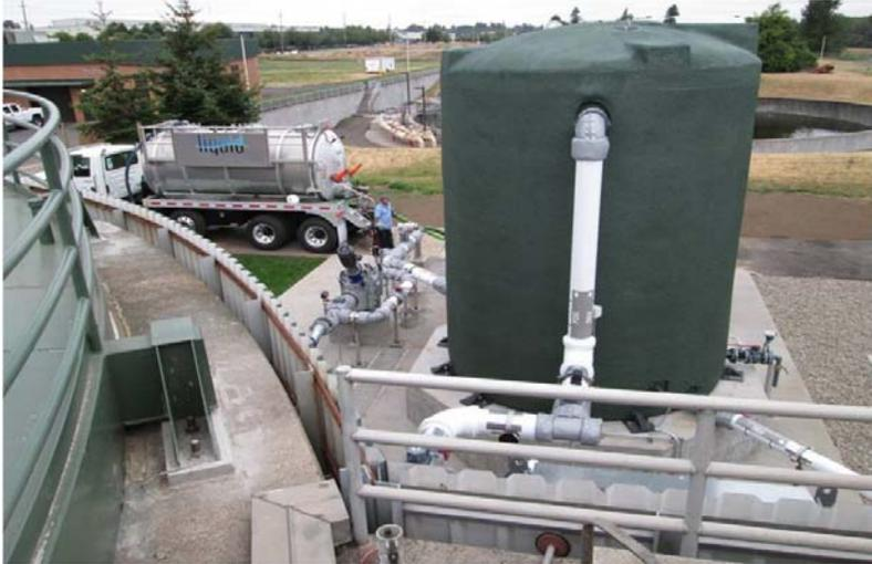
**Photo 1:** FOG Receiving and Feed System are designed to require no plant staff involvement.
