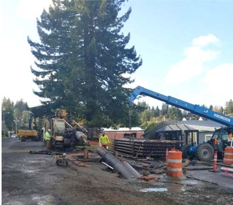
Photo: The HDD Rig and Entry Pit shown working around the Coast Redwood. In this photo, the conductor casing and 18-inch product pipe can be seen.
