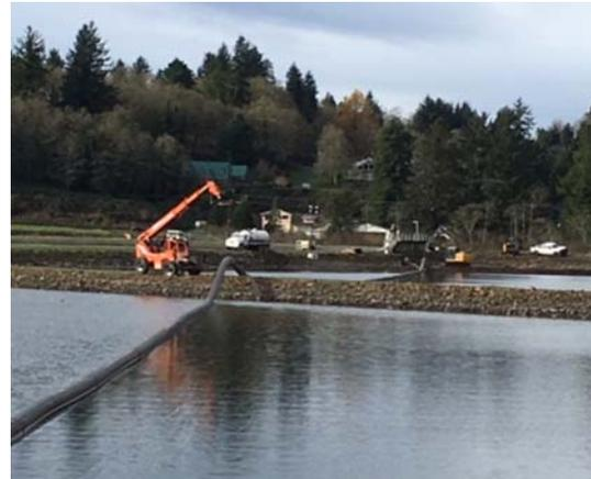
Photo: The HDPE pipeline shown lofted during pullback
