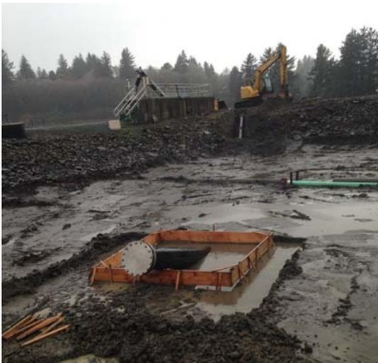
Photo: The exit pit with the pipeline installed and the headworks connection underway
